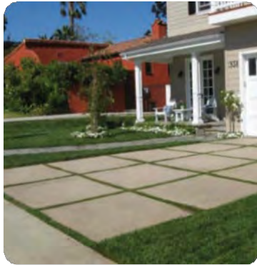
Permeable Paver Driveway Photo Credit: City of Los Angeles
